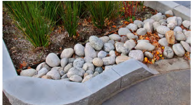
Rain garden used within a parking lot to reduce stormwater runoff.
