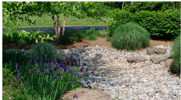
Bioswale alongside roadway.
