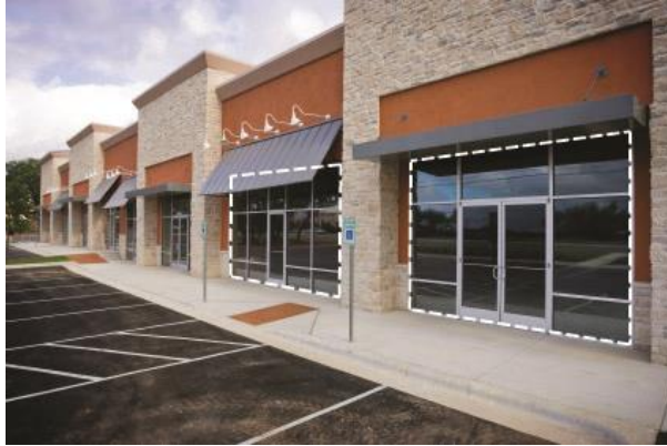
Figure 1127-F: The window area is illustrated within the dashed line area for the two storefronts in the above image.
