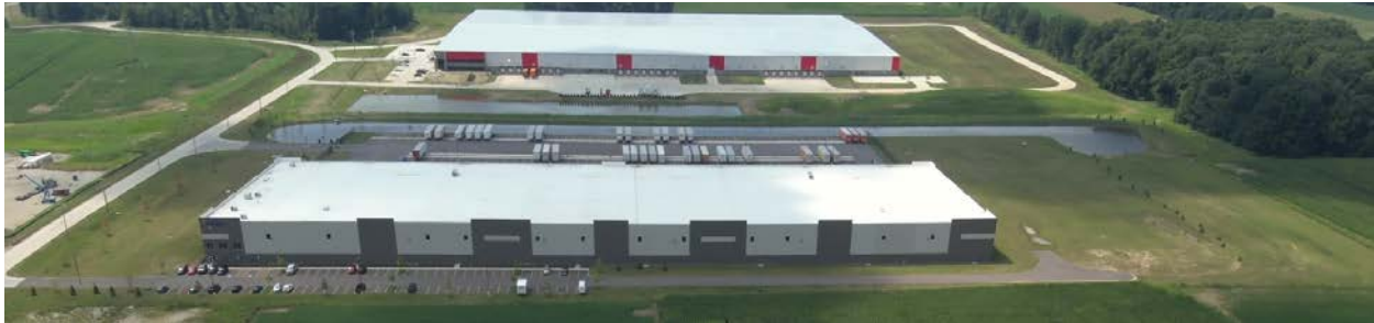
2023 Aerial showing the completion of the Wooster Brush & Frito-Lay expansions.
