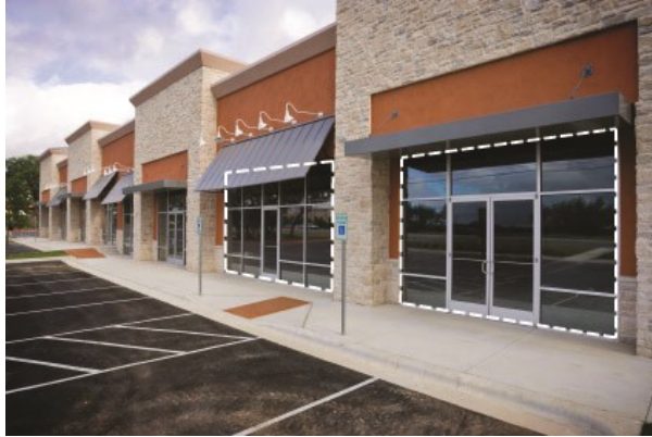
Figure 1127-F: The window area is illustrated within the dashed line area for the two storefronts in the above image.
