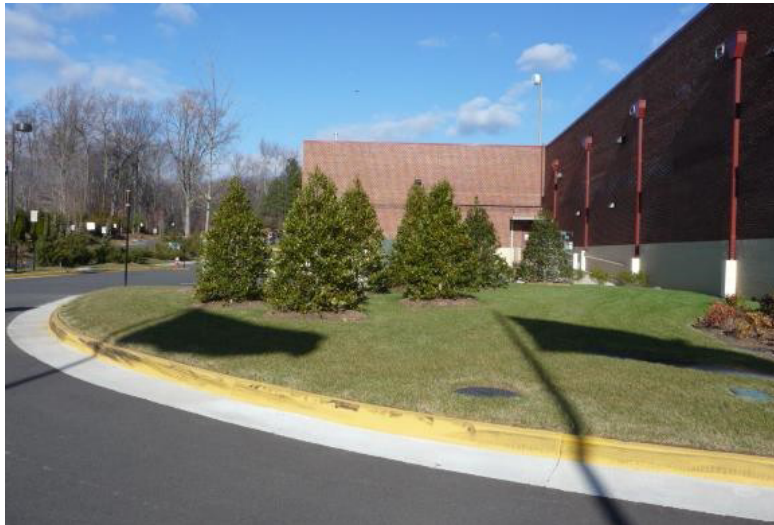
Figure 1123-C: The above image illustrates a vegetative screen that hides HVAC equipment and a dumpster.
