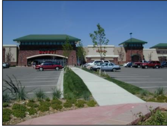
Figure 1125-C: This photograph illustrates how a sidewalk connecting the public sidewalk to the business can be integrated into the required landscaping.
