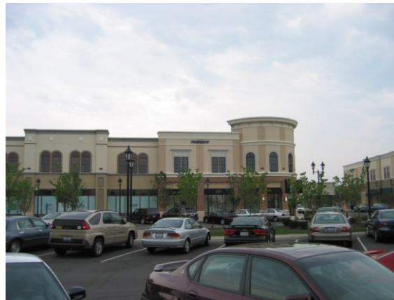
Figure 1119-G: Roofline changes shall be aligned with corresponding wall offsets and/or material or color changes.
