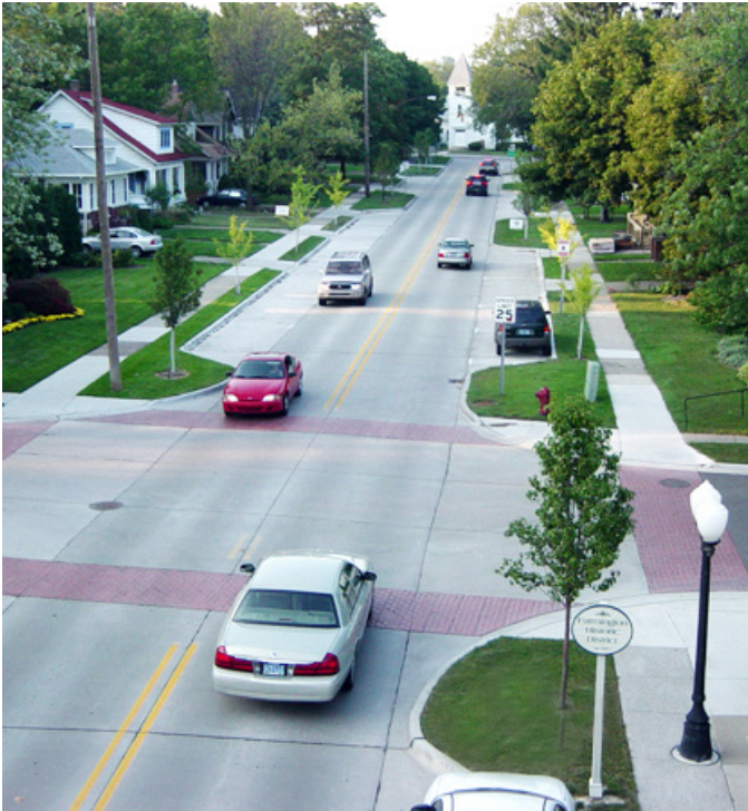
A "Complete Street" could see the addition of curb extensions, bricked crosswalks, signage and improved sidewalk conditions.
