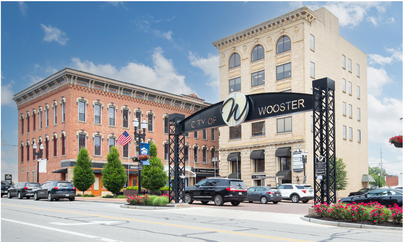
One of the methods used to gather information was a site visit and walking tour. The image above was taken on the walking tour and shows Wooster's downtown Center Green Park. This project was part of the 2015 Downtown Strategic Plan led by OHM Advisors.
