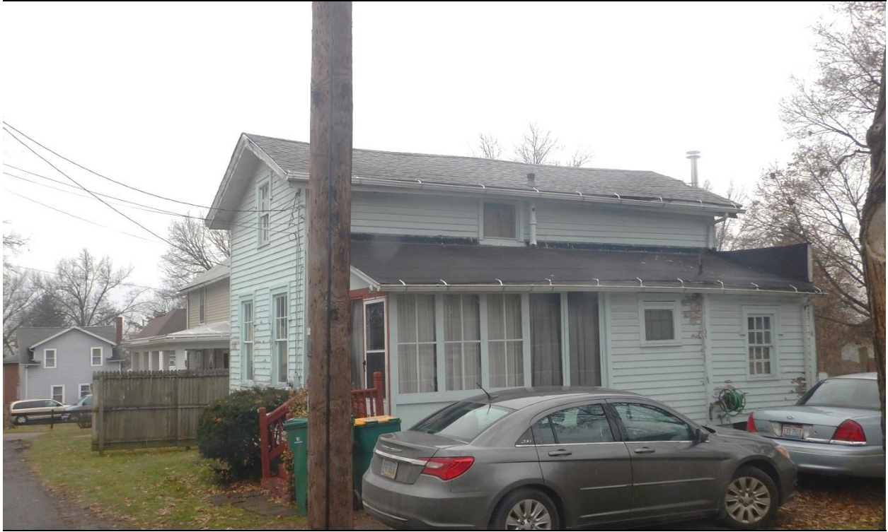
Disrepair: Bowing roofline, significantly exposed wood on exterior siding, rotting eaves.
