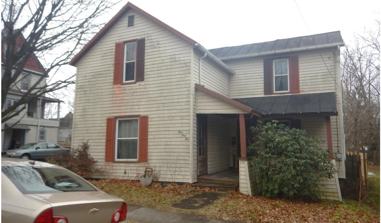
Disrepair: Porch floor caving in, rusting along metal roof. General disinvestment.
