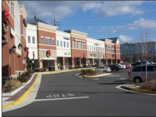
Figure 1119-H: Parapet walls with cornice treatments are used to disguise flat roofs. The image on the right illustrates a tall, thin parapet wall that is prohibited.
