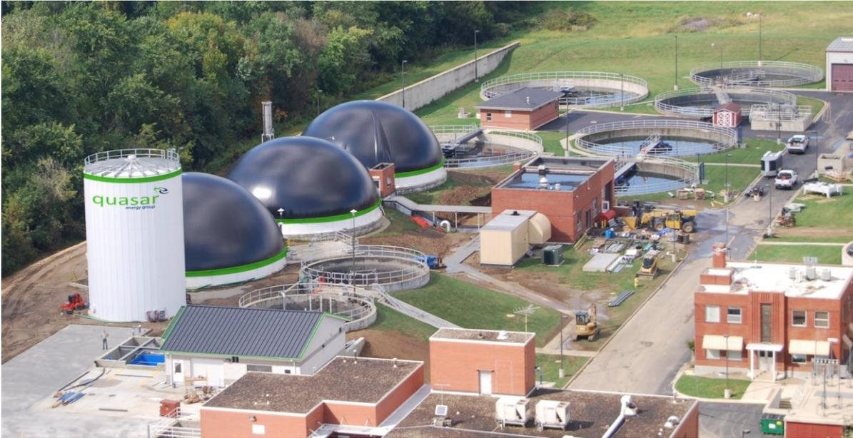
The “wet stream improvements” recommended in the 2012 URS Plant Evaluation Report, have been designed and the project will be released for bid in the summer of 2014. The Permit to Install has been submitted to the Ohio EPA and we are awaiting approval. Construction is slated to begin this year and completed by the end of 2015. The major components of the improvements are increased aeration, better scum removal (including fats, oil and grease), SCADA enhancements and clarifier rehabilitation.
