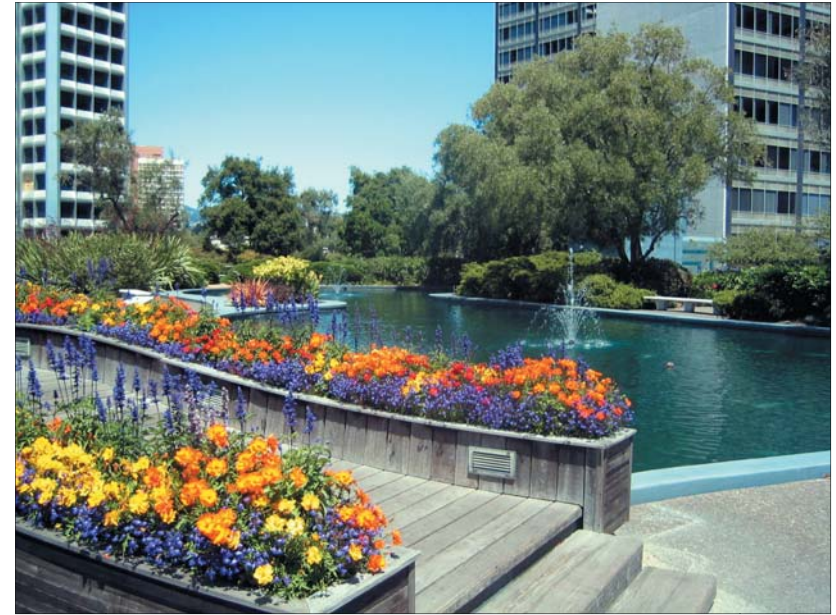
Figures 6-4: The Kaiser building, in downtown Oakland, illustrates how water storage and harvesting techniques may be used to irrigate intensive green roofs, increasing their stormwater benefit and reducing fresh water consumption.
