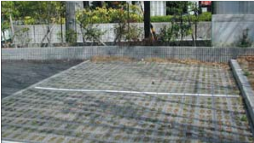
Figure 6-14: Permeable pavers may be appropriate in low traffic areas such as parking stalls.
