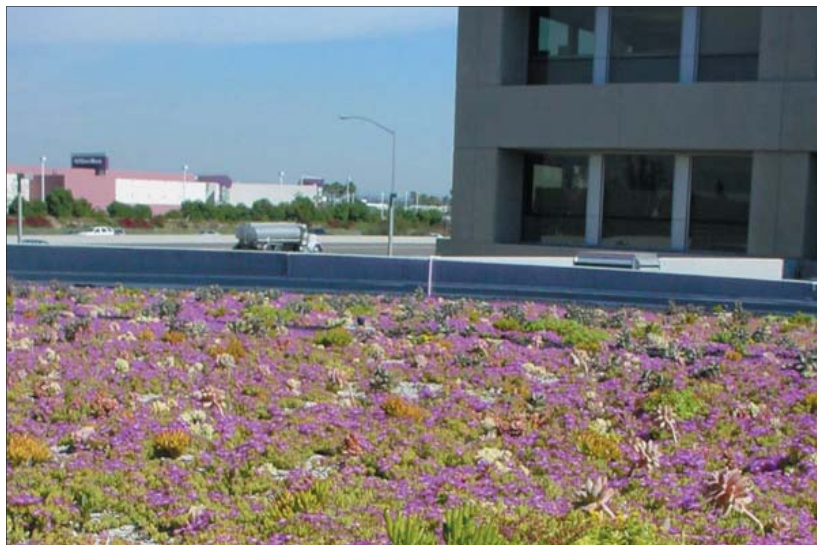
Figures 6-5 and 6-6: Extensive green roofs can thrive in a Mediterranean climate. The Gap Headquarters Building, in San Bruno, CA (top) and the Ford building, in Irvine, CA (bottom).
