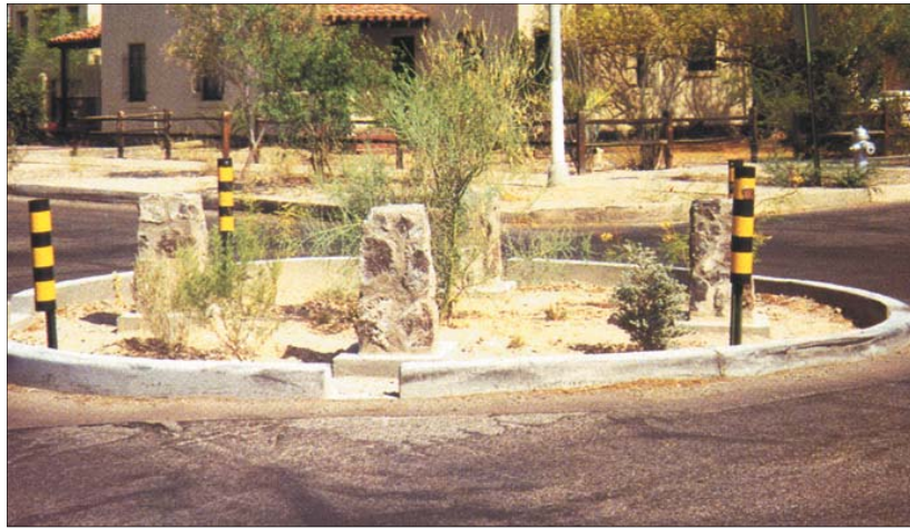
Figure 6-12: This infiltration basin doubles as a traffic circle.
