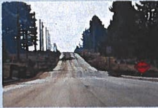
Melrose Drive Reconstruction Phase 2
