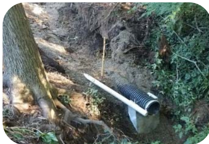
Beechwood Ave Storm Sewer Outlet Wenger Excavating
