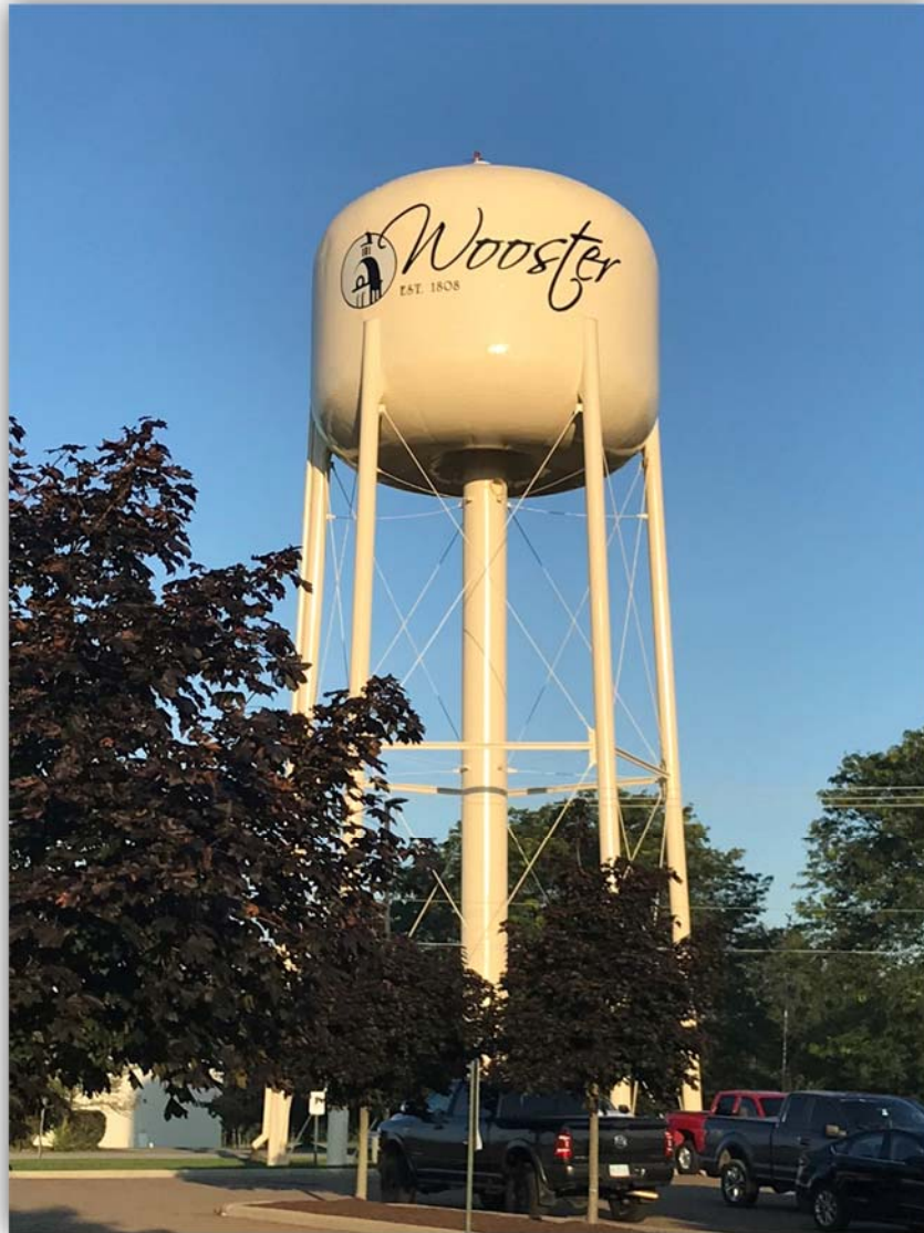
Industrial Park (IP) Water Tank Painting Project D & M Painting Corporation
