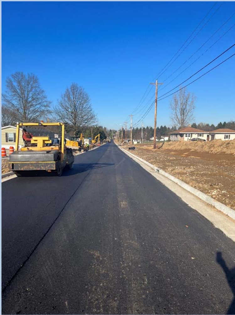
Melrose Drive Reconstruction Phase 2 Dirt Dawg Excavating, LLC
