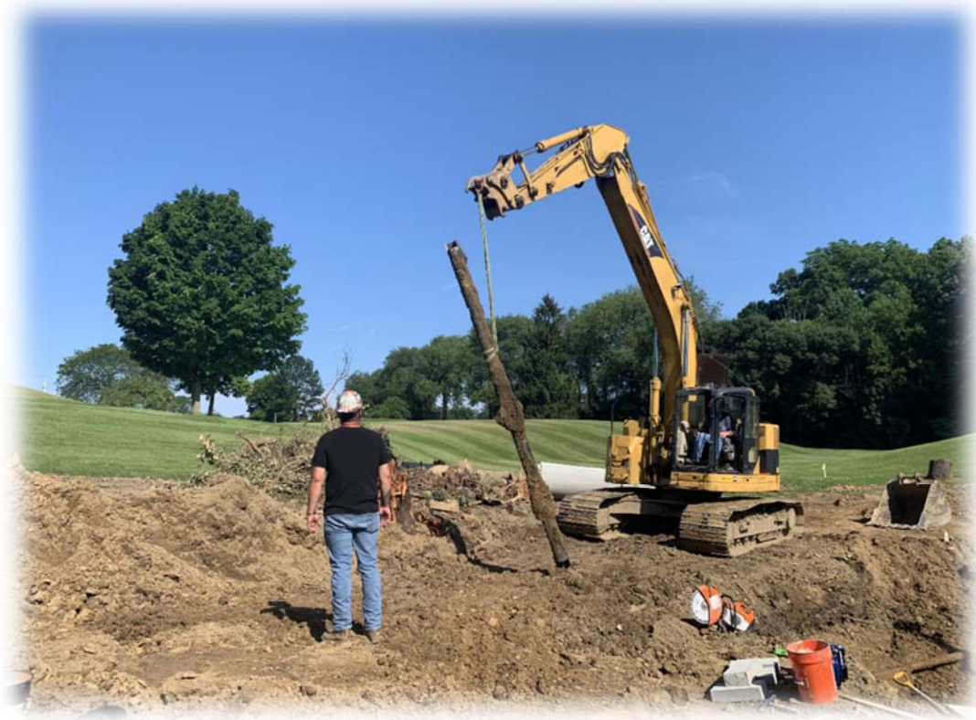
Palmer Street Culvert Replacement Boss Union Contracting, Inc.
